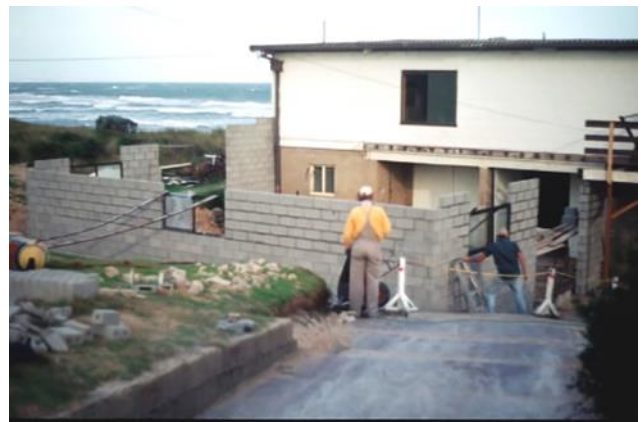
Original club driveway demolished to make way.
