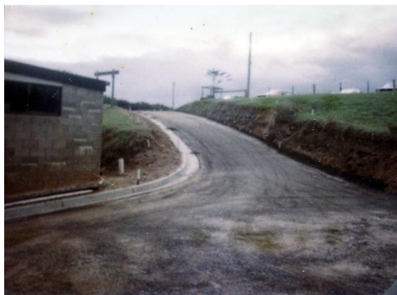
Above: The new bitumen driveway going in. A relief from the repeated clay floods into the gear store area.
