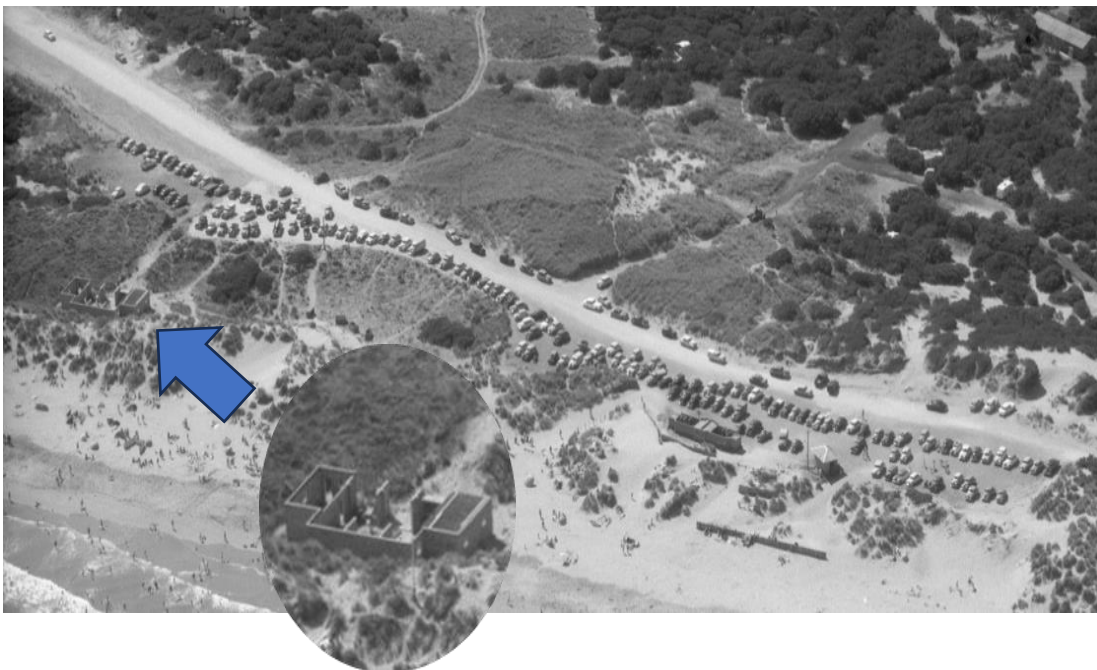
This photo (left) shows the clubhouse under construction around 1956/57.
