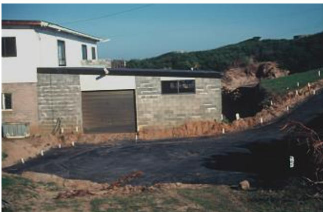
Above: The new bitumen driveway going in. A relief from the repeated clay floods into the gear store area.
