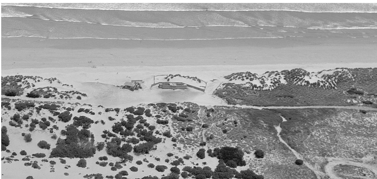
Ocean Grove main beach 1949. Ray's kiosk (left) and change rooms.
